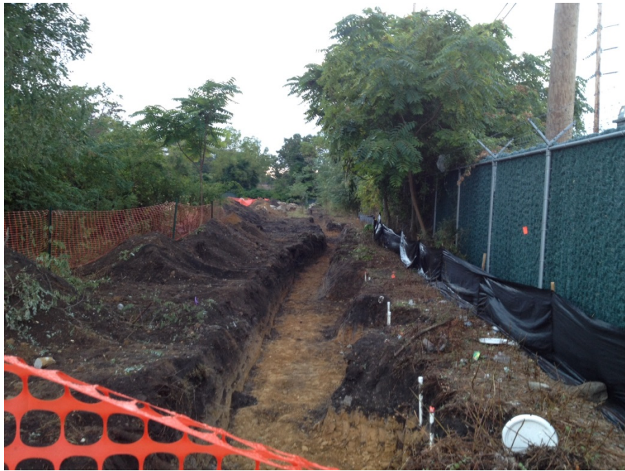
Excavated trench at 66 North Clinton Avenue
